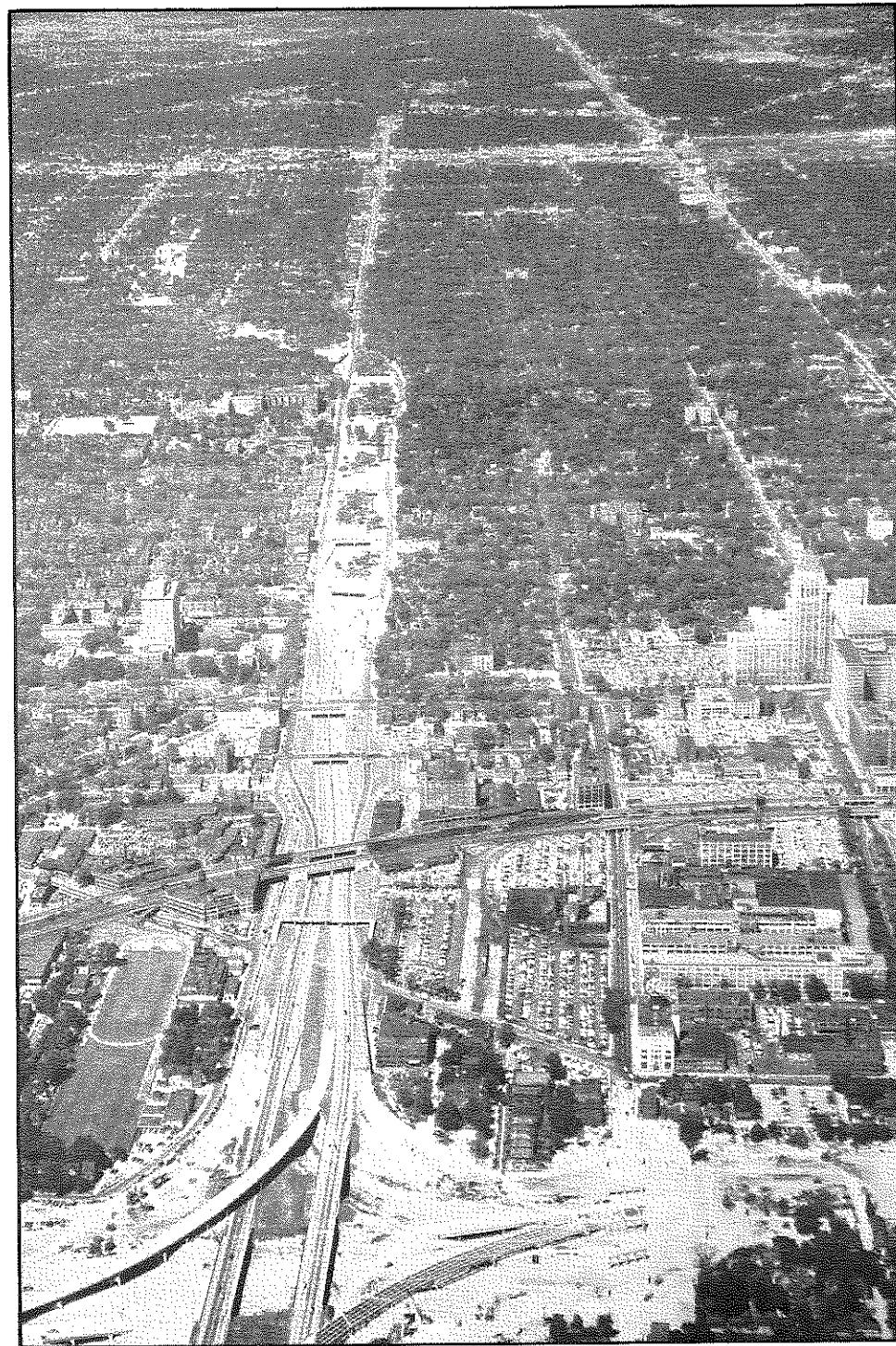
The John C. Lodge Expressway, northerly from the Ford-Lodge Interchange, showing the completed section and the portion under contract. The Fisher and General Motors buildings will be noted in the right center of the picture.
