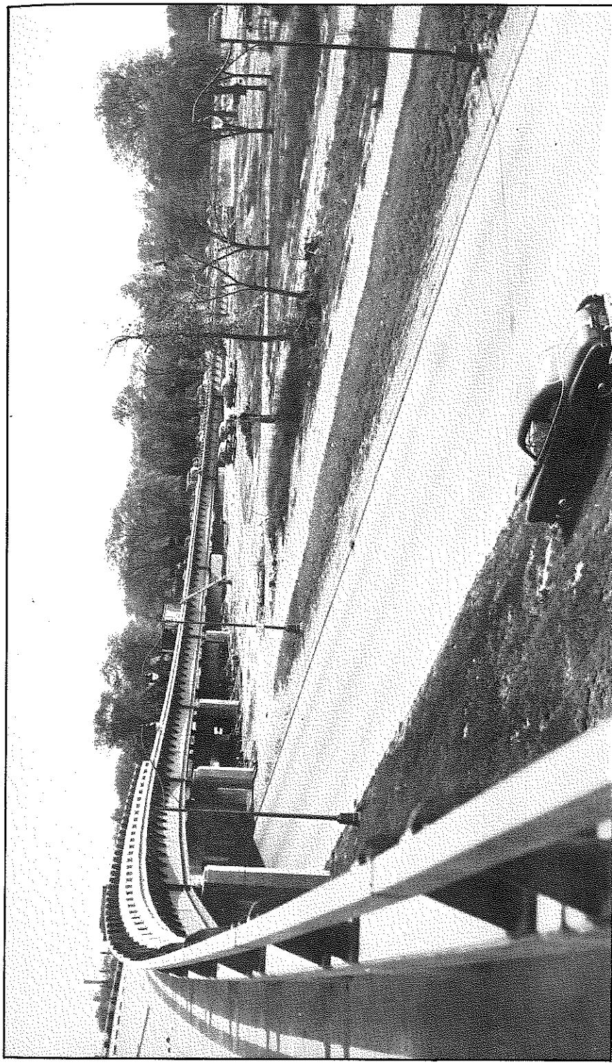
A close-up of a portion of the northwest section of the Ford-Lodge Interchange showing the ramp and structures which provide for eastbound traffic from the Ford Expressway to go north on the Lodge Expressway.
