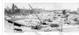
The 1-mile-long freeway broke ground in January 1959. Families living within the path of the Chrysler Freeway (Interstate 375, as well as businesses, were given 30 days to vacate upon receiving notice.
